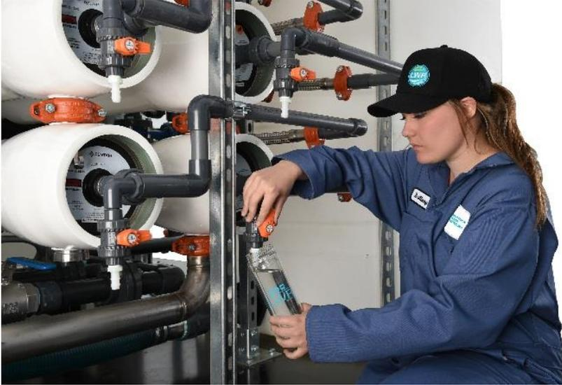
The LWR System segregates and concentrates livestock manure into nutrient rich solid and liquid fertilizers, while the rest is recycled into clean, potable water.
