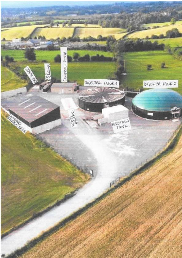
Par Biogas, a farmer owned anaerobic digester company in Northern Ireland produces renewable energy from silage and the slurry from livestock farming. They have been supplying energy to the National Grid since January of 2015.
